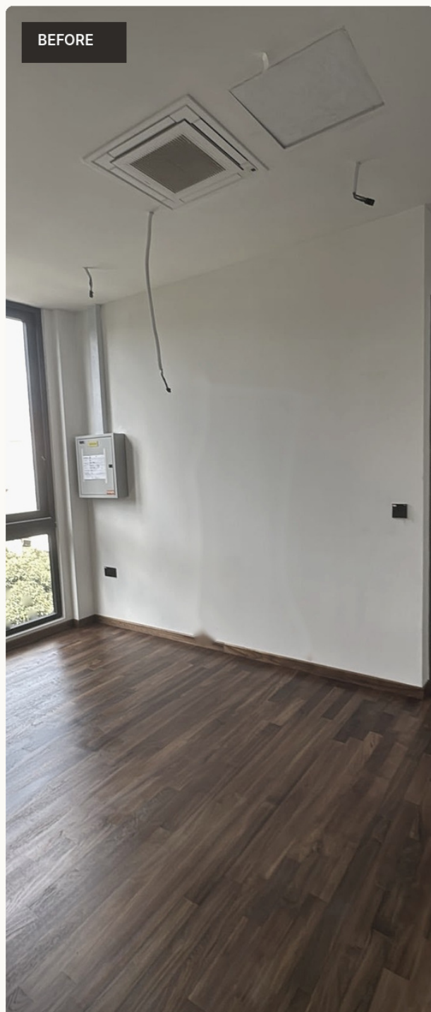
Clean shell / services in progress
